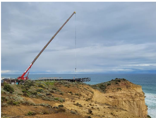
'Project Saddle Lookout' viewing platform being built at the Twelve Apostles
